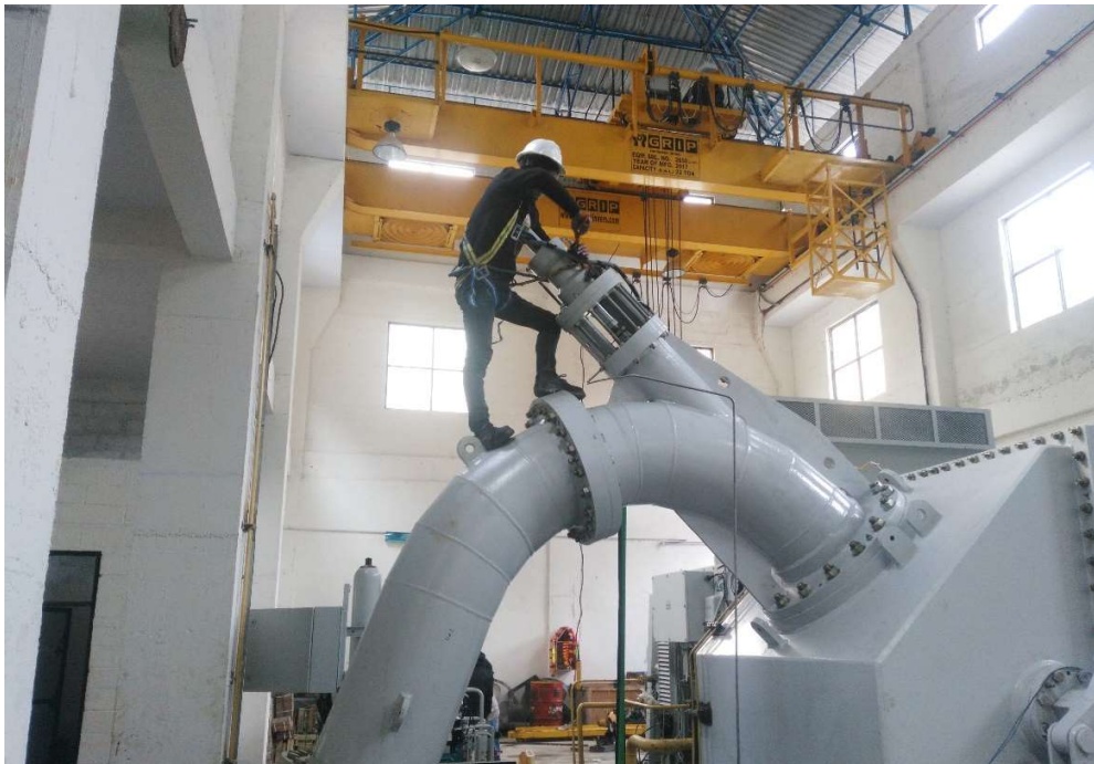
FIGURE 6 REAMING WORK ON BRANCH PIPE
