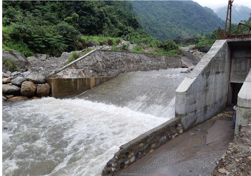
Fig Headworks completed view.
