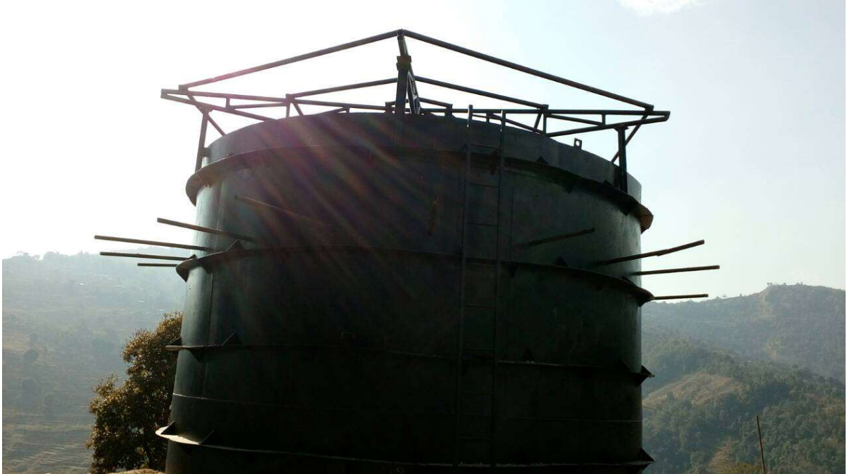
Fig : completed view of Surge
