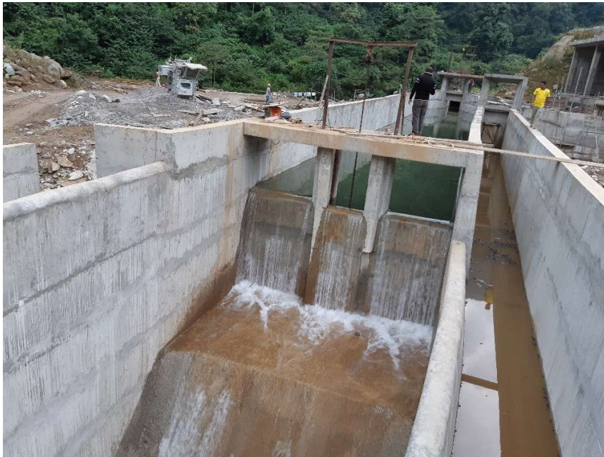
Fig 2: Water filling has started.
