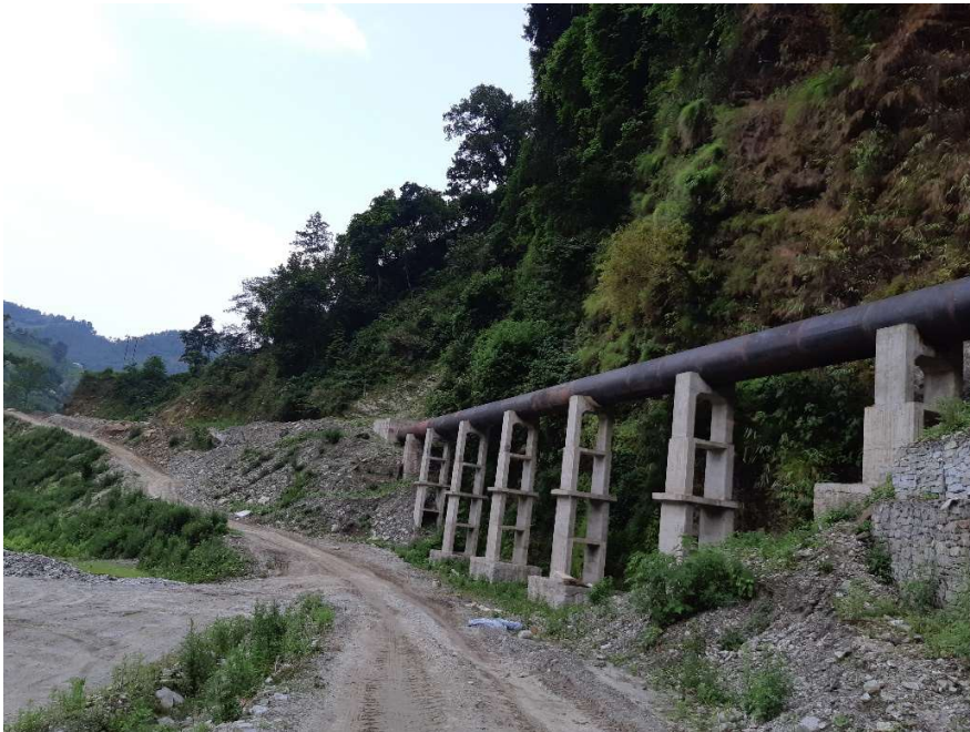
Fig 10: Headrace pipe section between AB-38 to AB-39
