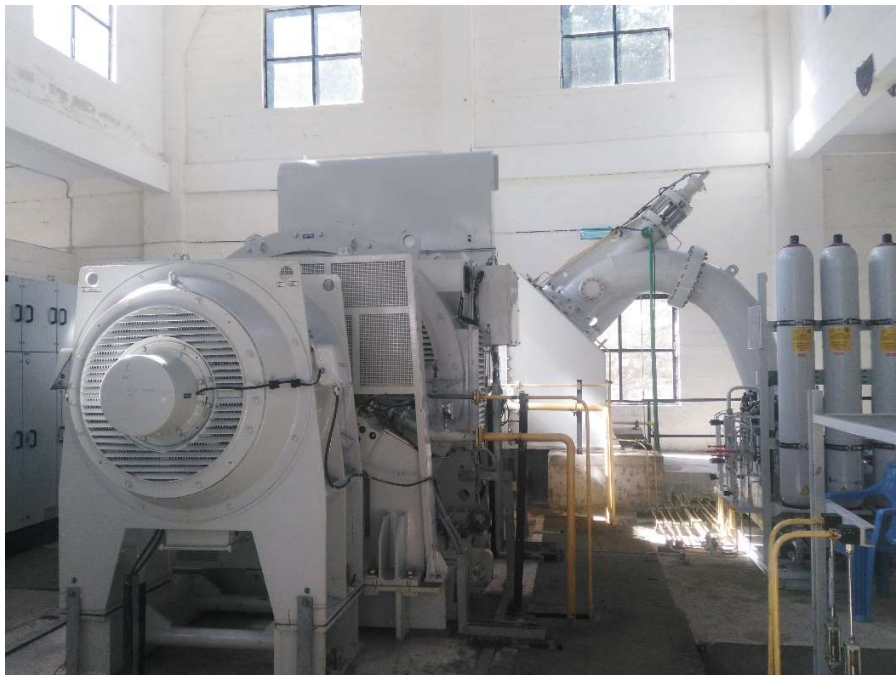
FIGURE 1 UNIT 2 AFTER COMPLETE ERECTION
