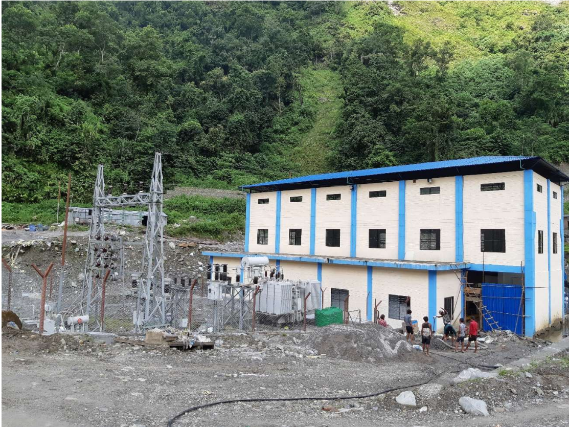
Fig15: Completed view of Rudi A Powerhouse.
