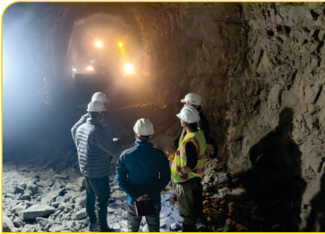
Khimti 2 HEP Adit 1 Tunnel
