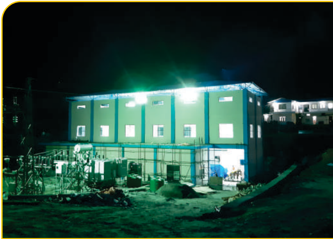
Rudi A Power house nightview
