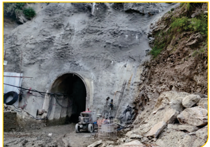
Khimti 2 HEP Headworks
