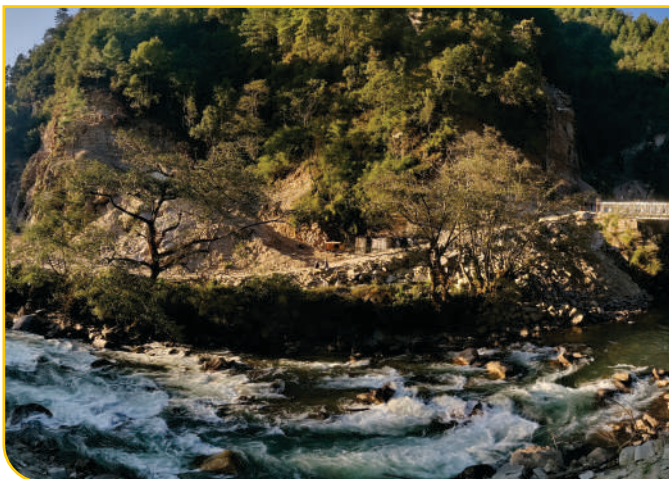
Khimti 2 HEP Headworks
