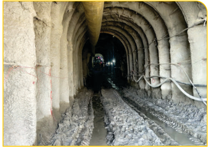
Khimti 2 HEP HRT Inlet Tunnel
